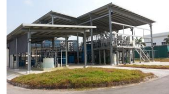
1,000 m 3 /day Integrated Validation Plant
